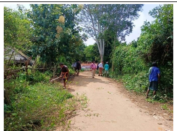
Cleaning of roadside bushes and trimming of unwanted tree branches
